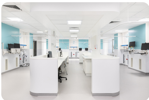
Images of theatres (top) and recovery (bottom) installation
